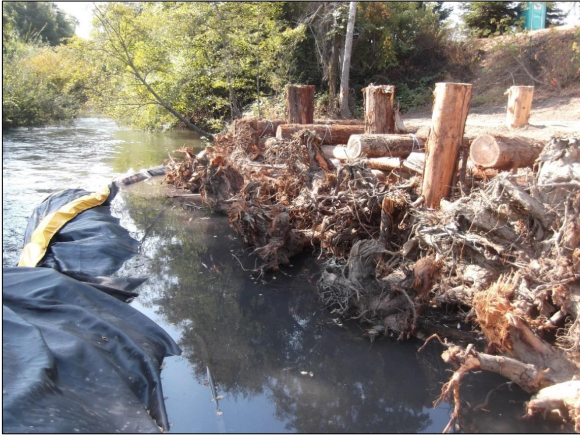
Figure 2-11 Log Revetment Immediately Post Construction
