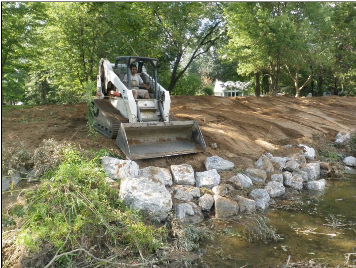
Figure 2-10 Rock Revetment Under Construction
